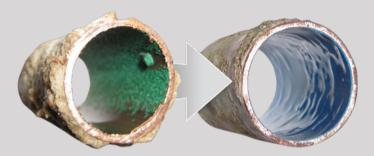
The AirKote® SLR process is utilized to install an internal NSF61 epoxy coating to leaking 1/2" through 1" copper and galvanized pipe sections up to 50' in length. The epoxy coating is listed by ICC-ES file# PMG-1749
